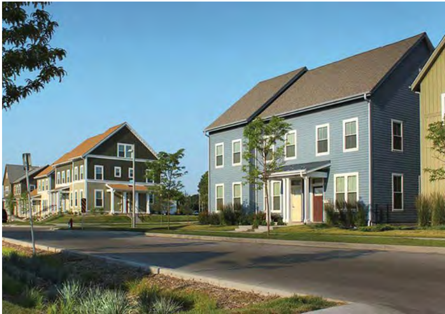
Figure 15 Multi-family residential complex at Westlawn Gardens in Milwaukee, Wisconsin illustrate what updated development standards can result in.
