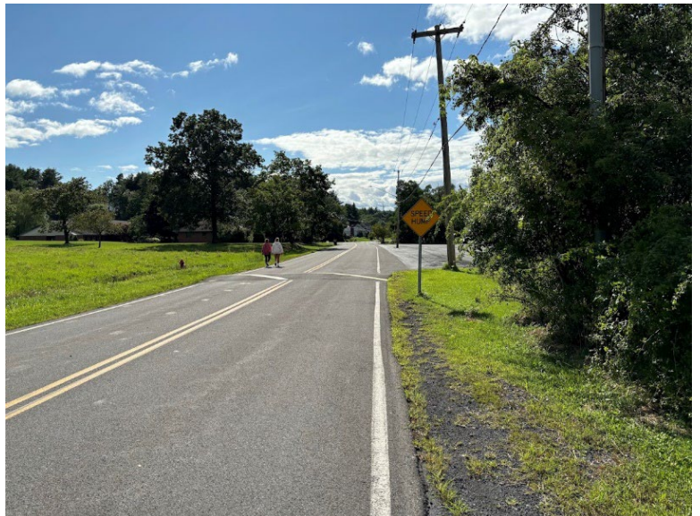
Figure 26 Speed Bump on Mountainview Street, Looking West
