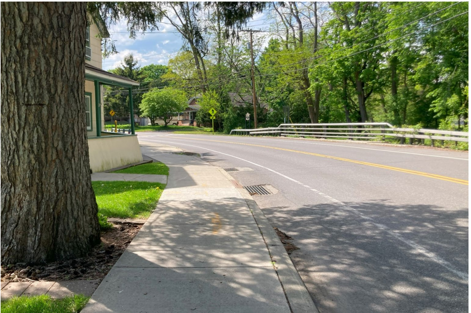
Figure 28 View of NYS-85A Mid-Block Crossing Existing Conditions
