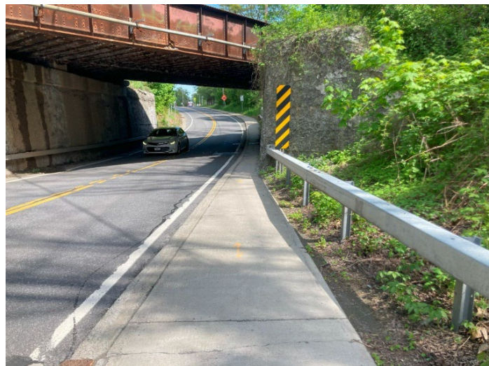
Figure 16 Narrow Sidewalks at CSX Railroad Underpass
