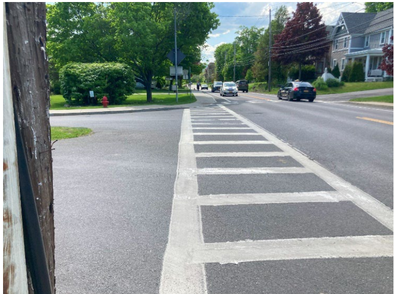
Figure 19 Pedestrian Crossing at Stonington Hill Road and NYS-85A Looking West
