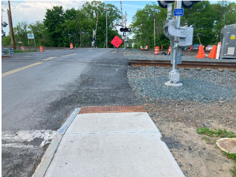
Figure 24 Terminus of Sidewalk on South Main Street and Missing Connection to North Main Street, Looking North
