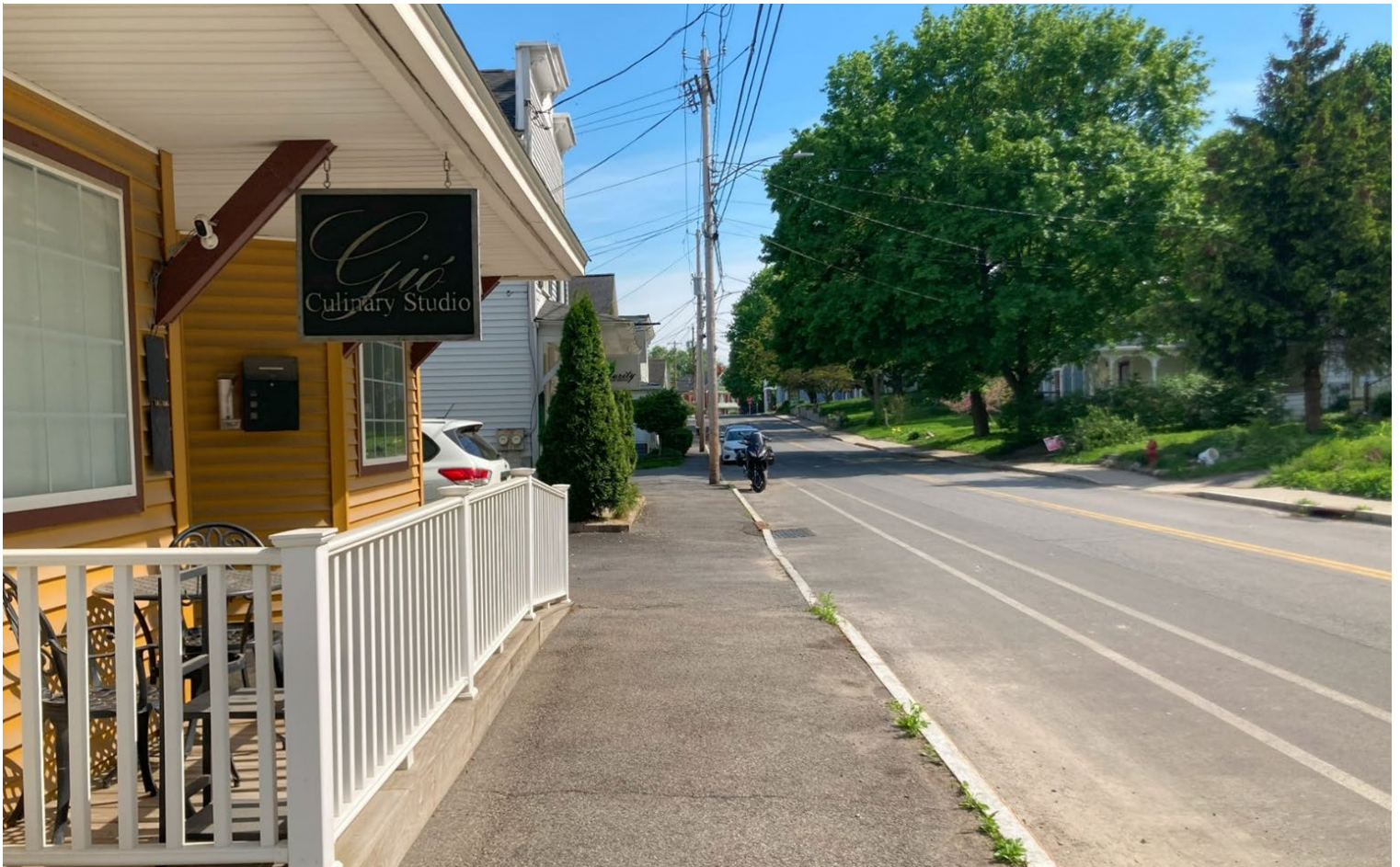
Figure 32 View of Current Sidewalk Conditions on South Main Street
