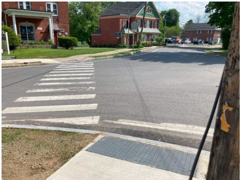
Figure 21 New Curb Cut Alignment, Intersection of Voorheesville Avenue and South Main Street, Looking South
